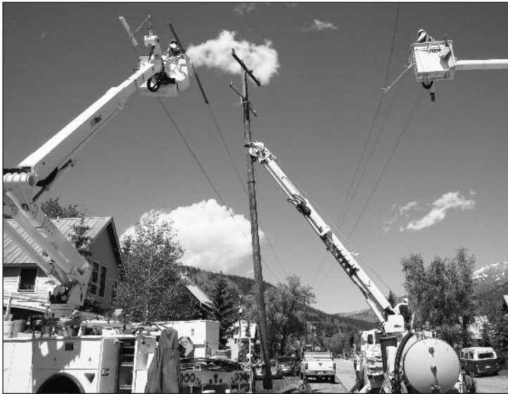
CPI begins Crested Butte Rebuild.
