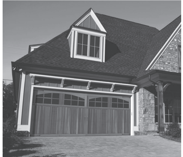
Garage doors add convenience and security to a home but should be routinely inspected.
