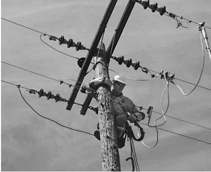
GCEA journeyman Ron Copenhaver takes safety precautions while working outdoors.
