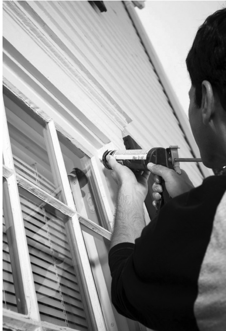
Sealing cracks around doors and windows can help save on your electric bill.
